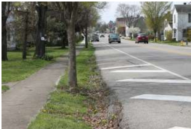
Figure 1.4 Example of Drainage Ditch in Downtown Bellbrook
